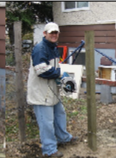
October 24 th @ 1415 Athol St. building the back yard fence. Great job!
